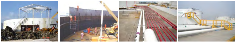
Tank construction, civil works and general installations - Poza Rica, Ver.
