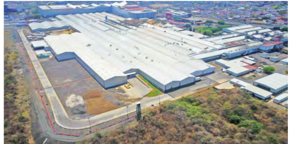
Warehouse Bridgestone Cuernavaca, Morelos.
