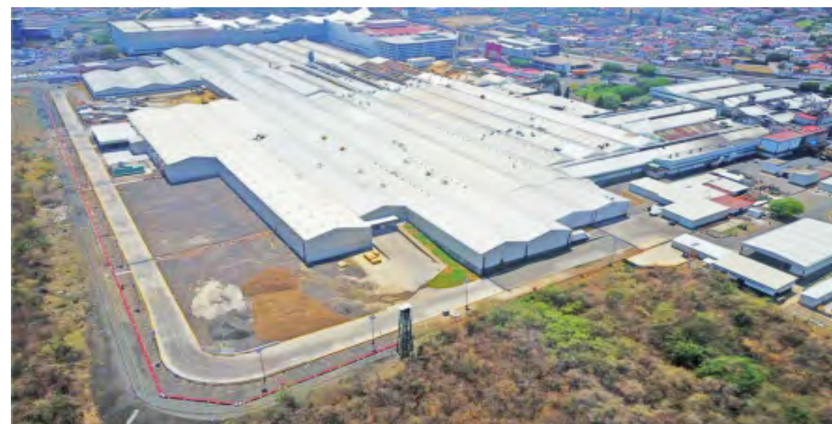
Nave Industrial Bridgestone Cuernavaca, Morelos.
