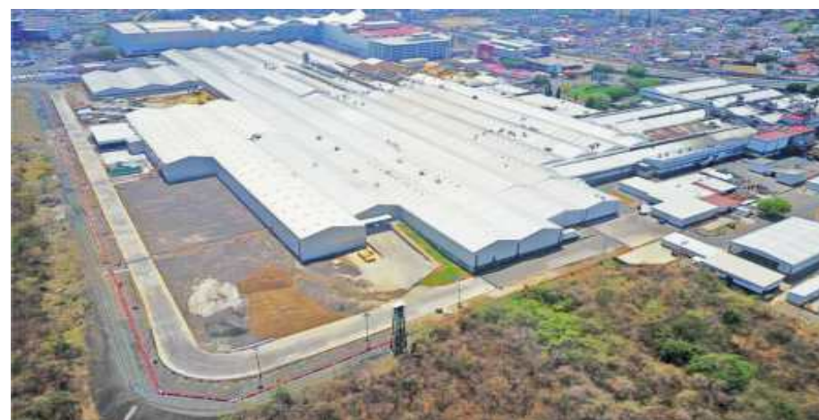
Nave Industrial Bridgestone
